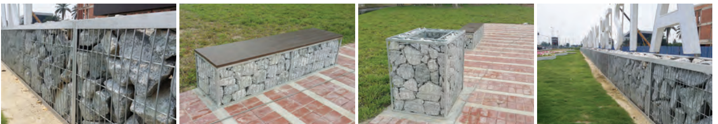
Feature Wall & Gabion Cage
